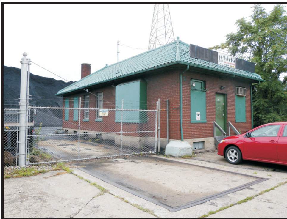
Plate A2. Former West Virginia Coal & Coke Company/Ohio River Company Coal Yard Office/ Scale House at 725 West Mehring Way, facing southwest.
