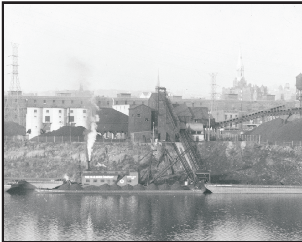
Plate A1. Ca. 1940 view of the south side of the West Virginia Coal & Coke Company/ Ohio River Company Coal Yard, facing north.
